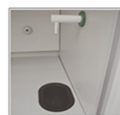
Water Tap & Water Sink
